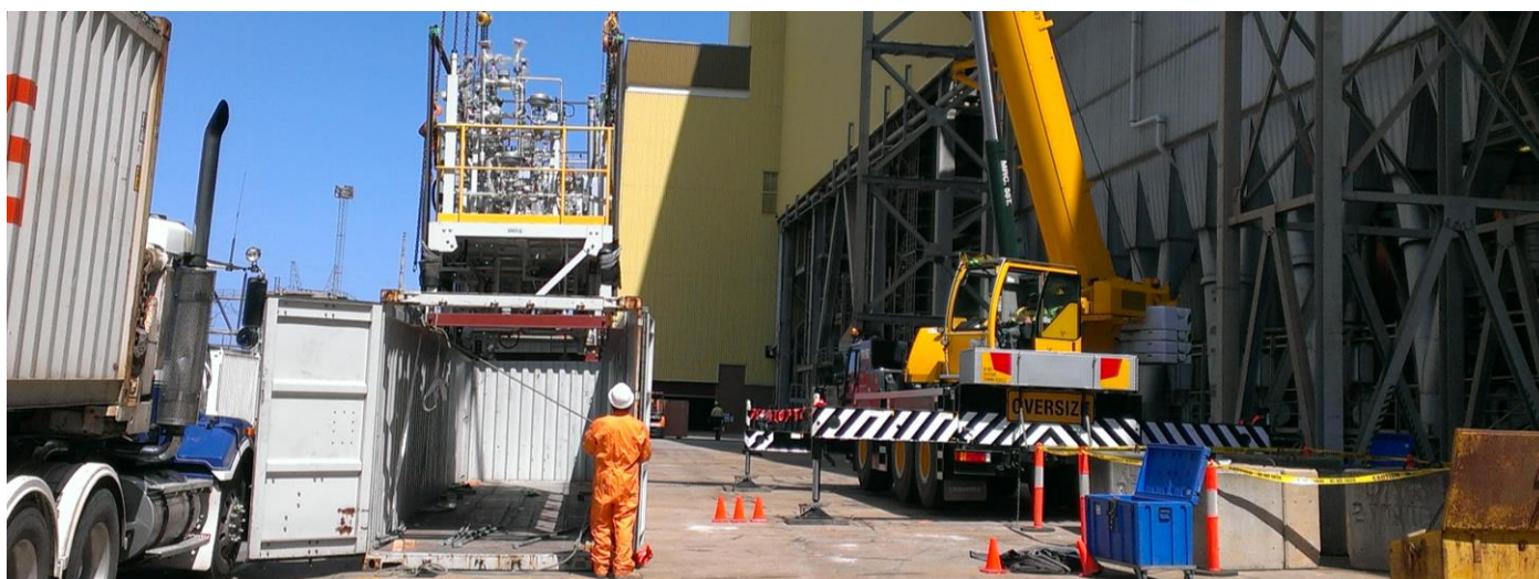
Figure 1: Unloading modules with crane (Copyright 2016, AGL).
