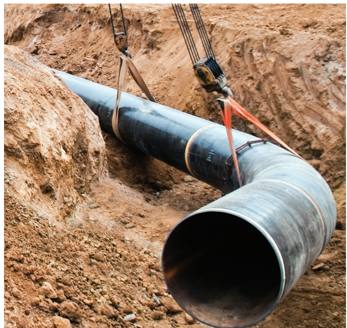
New CO 2 pipeline construction in US (3) .
